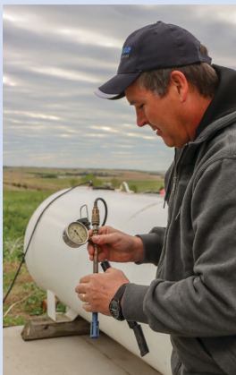
Lower Loup NRD Water Resources Technician Harold Benton inspects a check valve on a chemigation system in Valley County. Chemigation permit renewals in the LLNRD are due by June 1, 2026.
