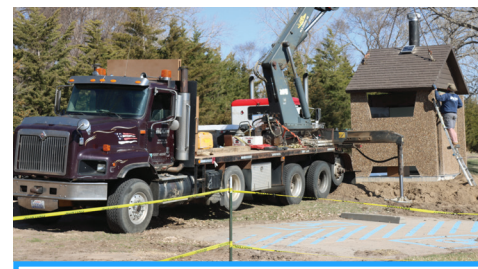
Restroom replacement at Pibel Lake.
