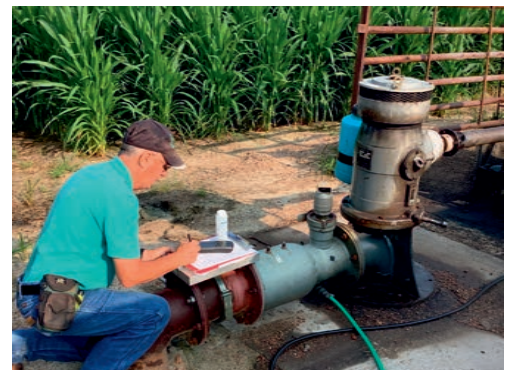
NRD Technician Dan Ray checks chemigation.
