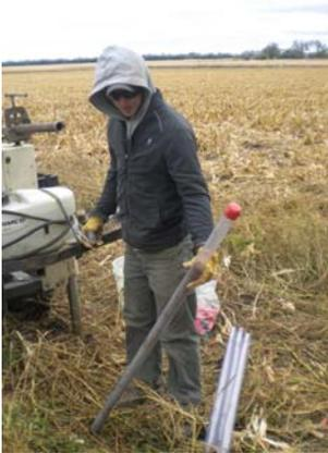
As dirt work is done for placement of a piezometer, core samples are saved for analysis of the geological components of the soil.
