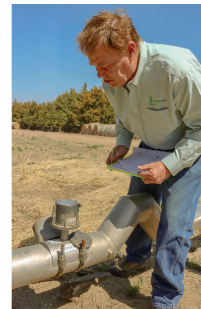
Lower Loup NRD technician Ed Drozd inspects a flow meter near Genoa
