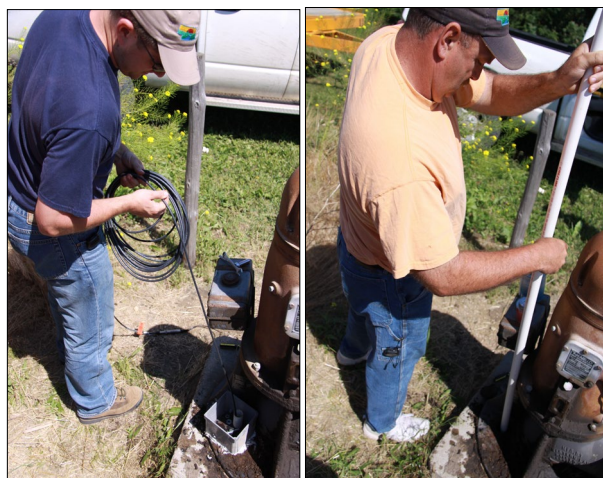
Irrigation Well – Boone County
